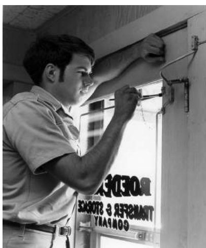
Dennis Maenhout installed door alarms at Roederer Transfer & Storage Company.
